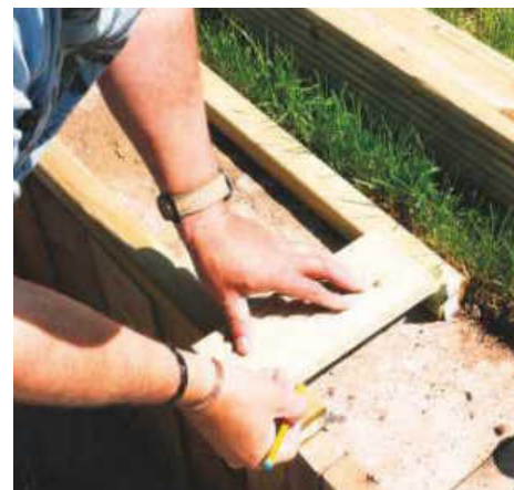
STEP 1. Using the spindles as legs, set out the width required and mark the deck board to length
